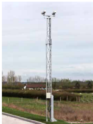
Altron Lattice Tower
