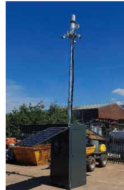
Dual Solar Panels on Tower
